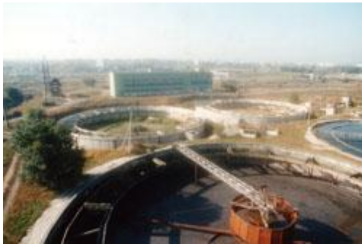
Figure 2. Chisinau Wastewater Treatment Plant
