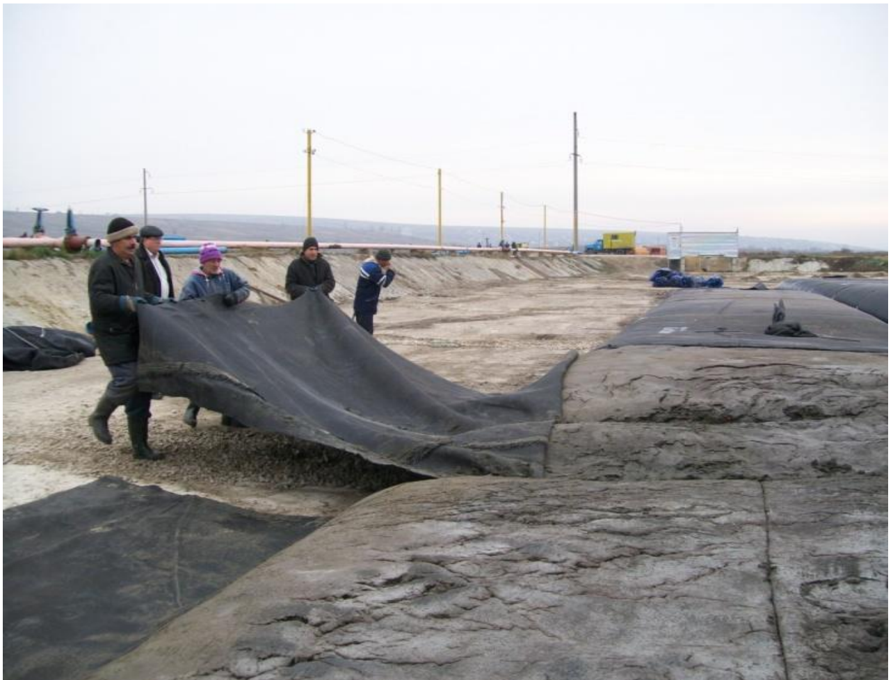
Figure 12. Opening of geotextile bags at Chisinau Wastewater Treatment plant
