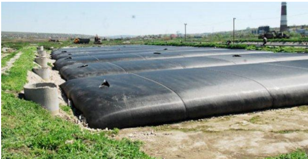
Figure 10. Geotextil bags from Chisinau Wastewater Treatment Plant
