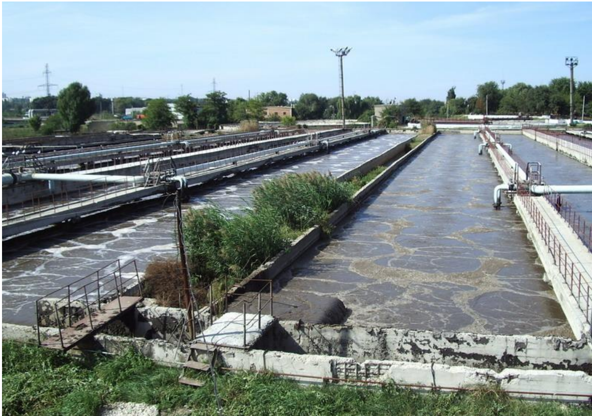
Figure 9. Aerated tanks with activated sludge
